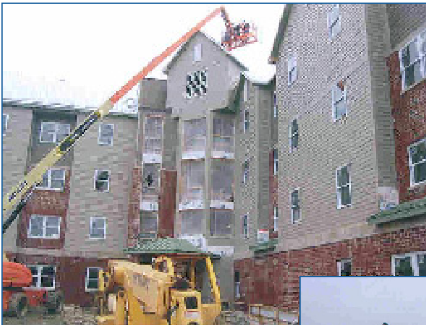
Employees using the boom lift
